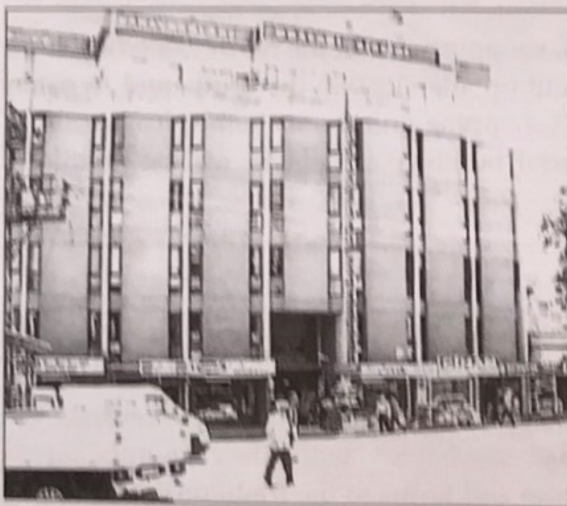
(Fig. 3a) Hasan Baba Building dominating the historic saele
