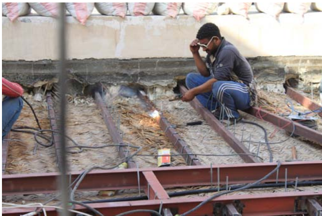
Fig. 9 Insertion of steel structures into traditional techniques of construction
