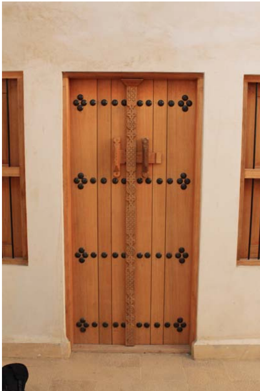
Fig. 4. Loss of patina through insensitive restoration applications
